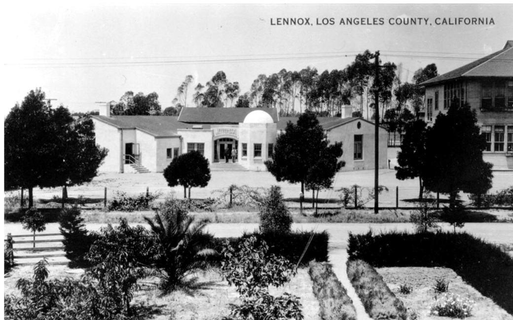
Jefferson School District Building Circa Early 1900's
